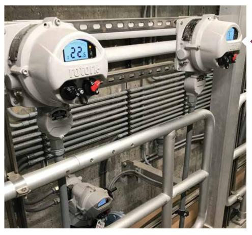
In the gravity filter plant, 18 butterfly valves are situated in an area beneath a walkway which made it difficult to access and operate the old actuators. With the new Rotork actuators, the installation of Remote Hand Stations (RHS) has now eliminated this problem.
