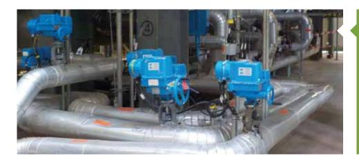
BLOWDOWN VALVE INSTALLATIONS WITH OLD ACTUATORS AT SSE GREAT ISLAND PRIOR TO THE UPGRADE.
