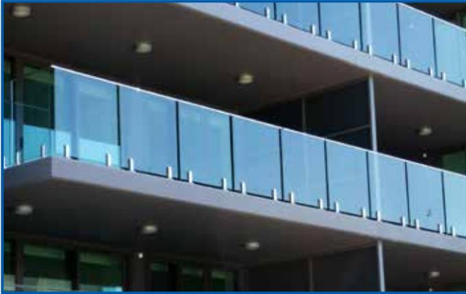
Spigots have been developed with our revolutionary tilt-lock adjustment technology to cover all loading requirements and glass thicknesses. Made from ultra-marine stainless Duplex 2205, these spigots are stronger and require less cleaning than Type 316.
