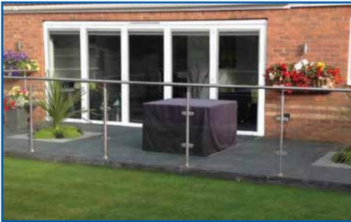
Satin polish pre-assembled glass clamp posts come in both  $\text{\O} 42.4$  and  $48.3\text{mm}$ , Type 304 and 316 stainless steel. End, corner and mid posts cut installation time dramatically to create a stylish glass handrail, made for 10mm glass, other size rubbers available.
