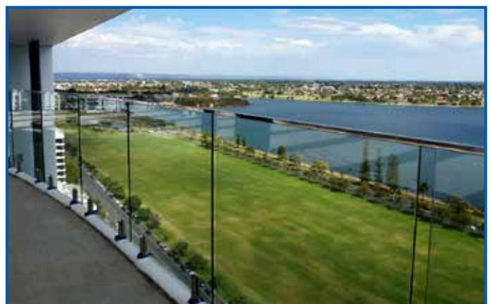
This system has been designed to reduce visual impact on top rail. Available in either round or square, stainless steel Type 316, all products are satin finish. Mini top rail is designed to suit 10 - 12mm glass and requires no welding.
