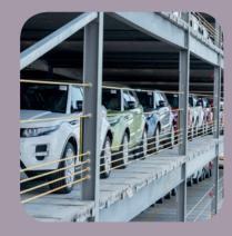
is a crucial one and in this instance Morgan Sindall selected the wire rope solution from Berry Systems. This deck is a steel framed construction with concrete slab decks and is the second deck at Southampton to have been fitted with Berry Systems' barriers. The standard Berry Brisafe system consists of 3 tensioned wire ropes running through a mesh panel that provides an integrated anti-climb feature and pedestrian handrail.
