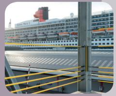
higher, fifth and sixth wires are at handrail height (minimum 1100mm) and complete the barrier by providing personnel protection. All wires were coated in bright yellow plastic for high visibility.
