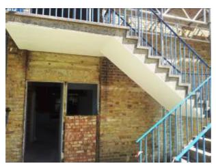
Apolodor used the same repair technique on the staircase using **RonaBond HB40**, the underside of the staircase was then jet washed before the application of white **RonaBond Crack Bridging Anti-Carbonation Coating WB**.
