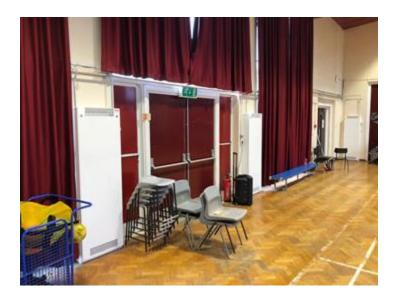
The classrooms posed its distinctive challenges with windowsills. The school replaced their old cast iron radiators with triple thin radiators that were made bespoke to fit each unique space.
