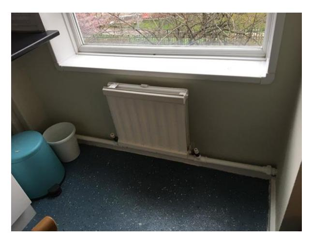
Prior radiators at this care home had exposed piping, this can reach up to a staggering 80°C. This provides potential dangers to the vulnerable individuals at the care home and doesn't align with safe surface heating guidelines.
