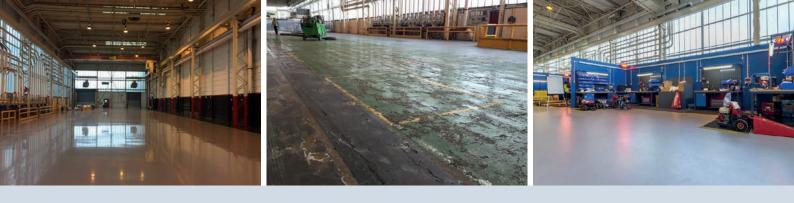
Therefore Zenith turned to UZIN for a specification. Zenith first utilised FM 30 industrial top in conjunction with RR 201 fibreglass reinforcement. This provided a loosely laid mesh that dispersed into the industrial top when laid, ensuring the strength and characteristics necessary to work on the asphalt substrate and providing a suitable base for the resin finish.
