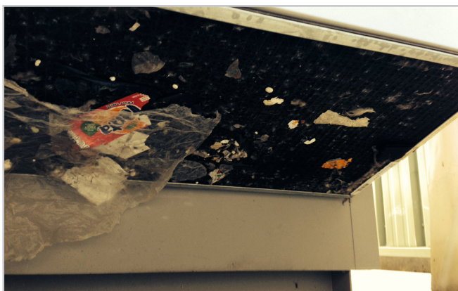
AHU Air Intake after two weeks
