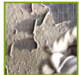
The above units are protected with a **RABScreen®**. This debris would have contaminated the equipment but is now kept on the outside where it can be easily cleaned off with a hose, brush or vacuum. A low impact on airflow with a high particulate capture from this electrostatic filter
