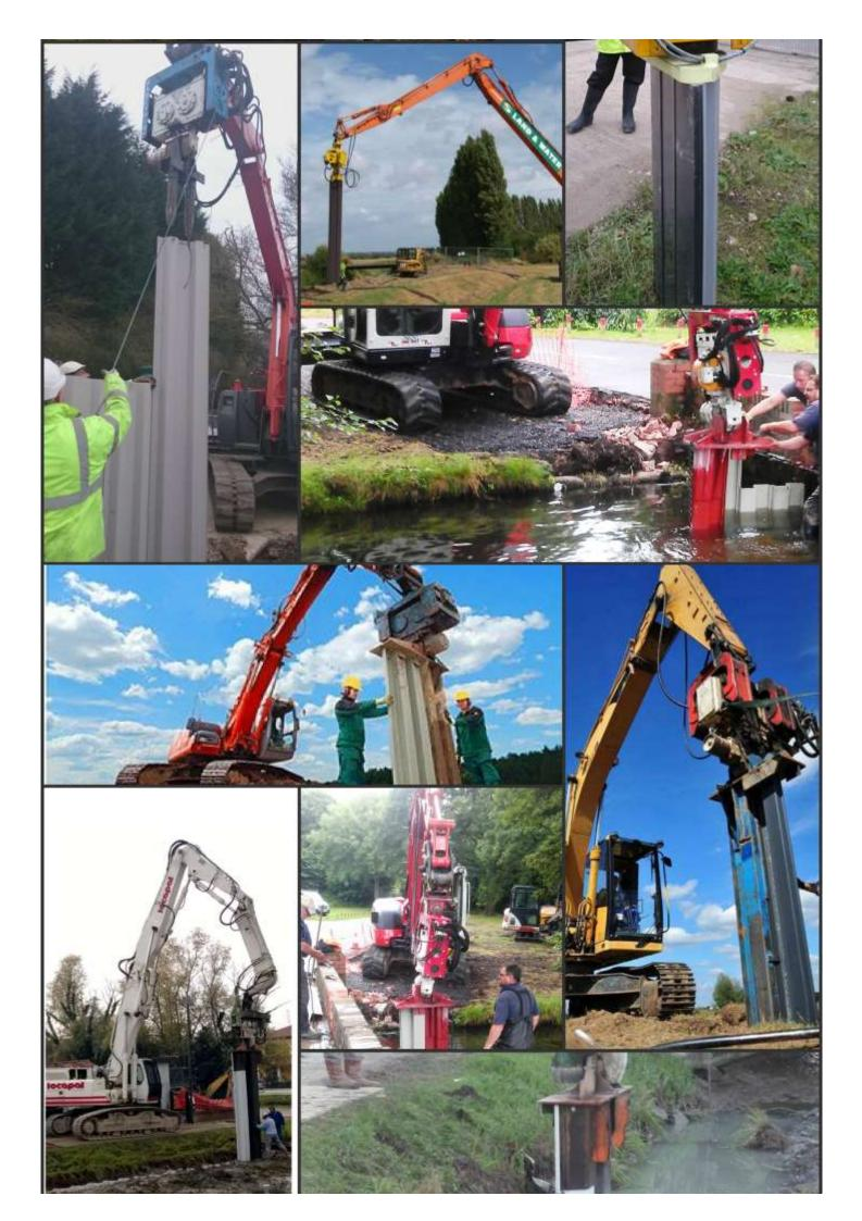
In terms of cold weather installation, PVC is quite resilient, but as the temperature drop below minus 5°C, care needs to be taken to prevent damage to the piling. A temperature of around minus 10°C is often stated as the limiting temperature for installation. It is advisable to consider thicker plastic piling, such as the Ultra Z11 in very cold working conditions.
