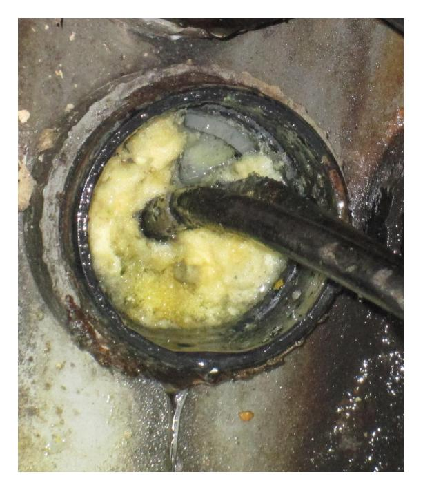
A typical Installation using expanding foam from a can. This will always **FAIL**.
