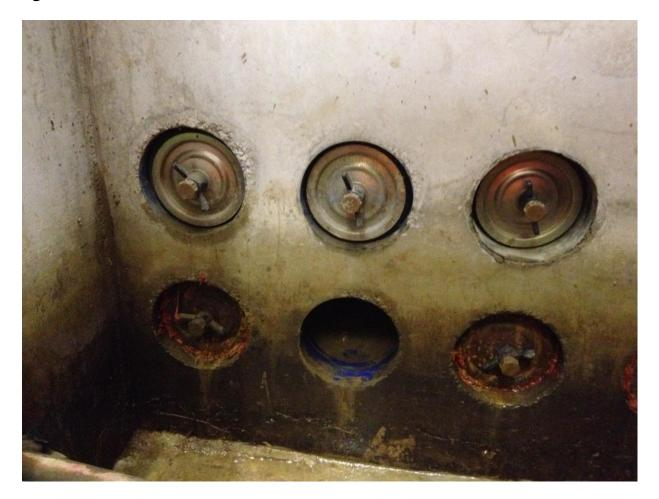
Illustrated on the left are temporary bungs that for whatever reason are allowing water penetration and corroding badly.
