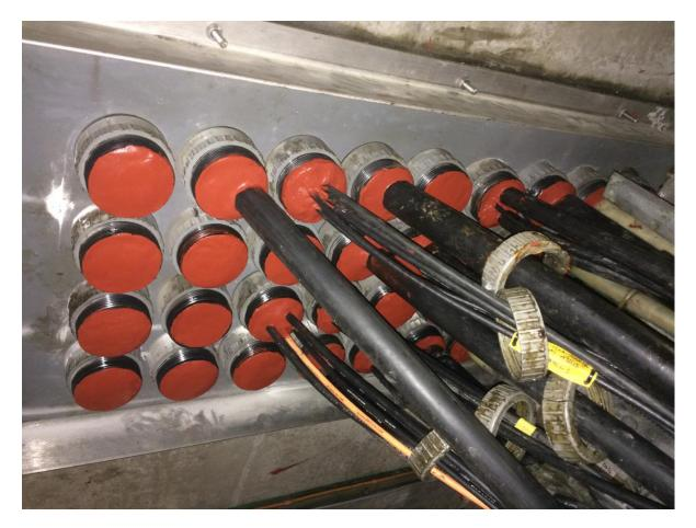
*FiloSeal+HD* is very easy to apply regardless of the type of cable scenario in the ducts as it uses strong, but flexible hexagonal tubes to support the cable and provide a strong backing for the seal.
