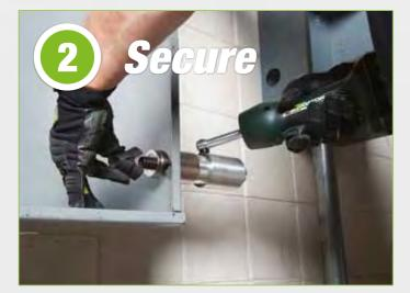
Secure SPEED LOCK onto draw stud: Faster setup and disassembly.
