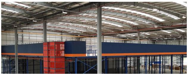
If you're not a hundred percent sure as to <u>what a mezzanine floor is</u>, it's a semi-permanent structure that creates an additional layer in between a part of your actual floor and the ceiling, making more storage space appear out of thin air (literally).
