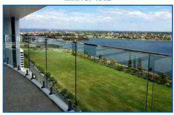
This system has been designed to reduce visual impact on top rail. Available in either round or square, stainless steel Type 316, all products are satin finish. Mini top rail is designed to suit 10 - 12mm glass and requires no welding.
