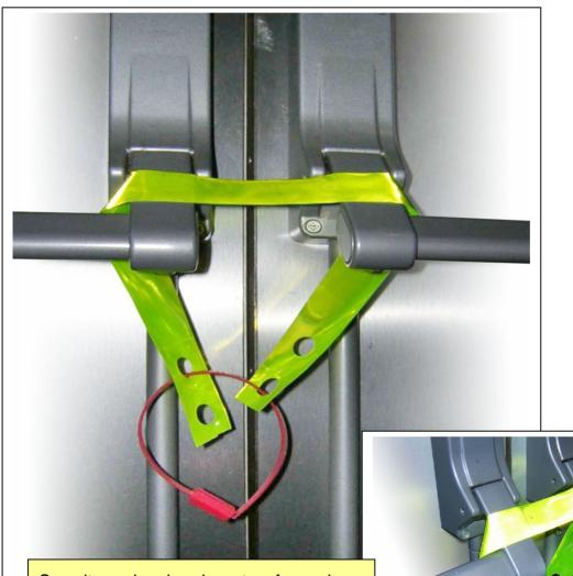
Security seal and sash system for push bar type emergency exits.
