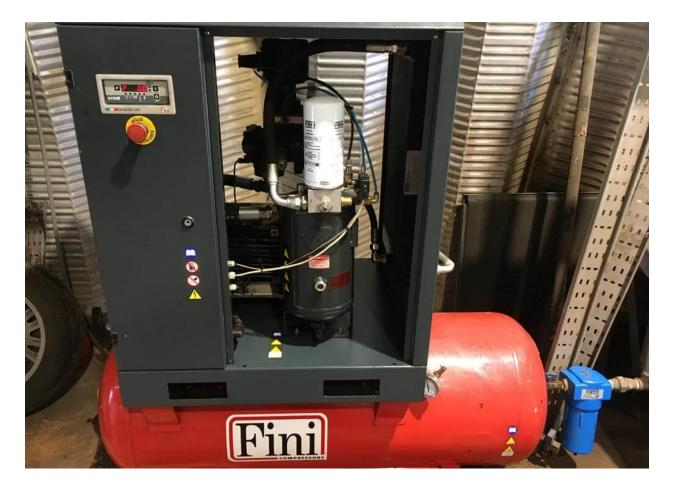
**Inefficiency**: Recently, we were called out to a Fini Quadro compressor which hadn't been serviced for years. It was still limping on, but our engineers found cracked drive belts that could have snapped at any moment, and leaking hoses that were wasting air, forcing the client to crank up the power in an effort to get more pressure to the tools.
