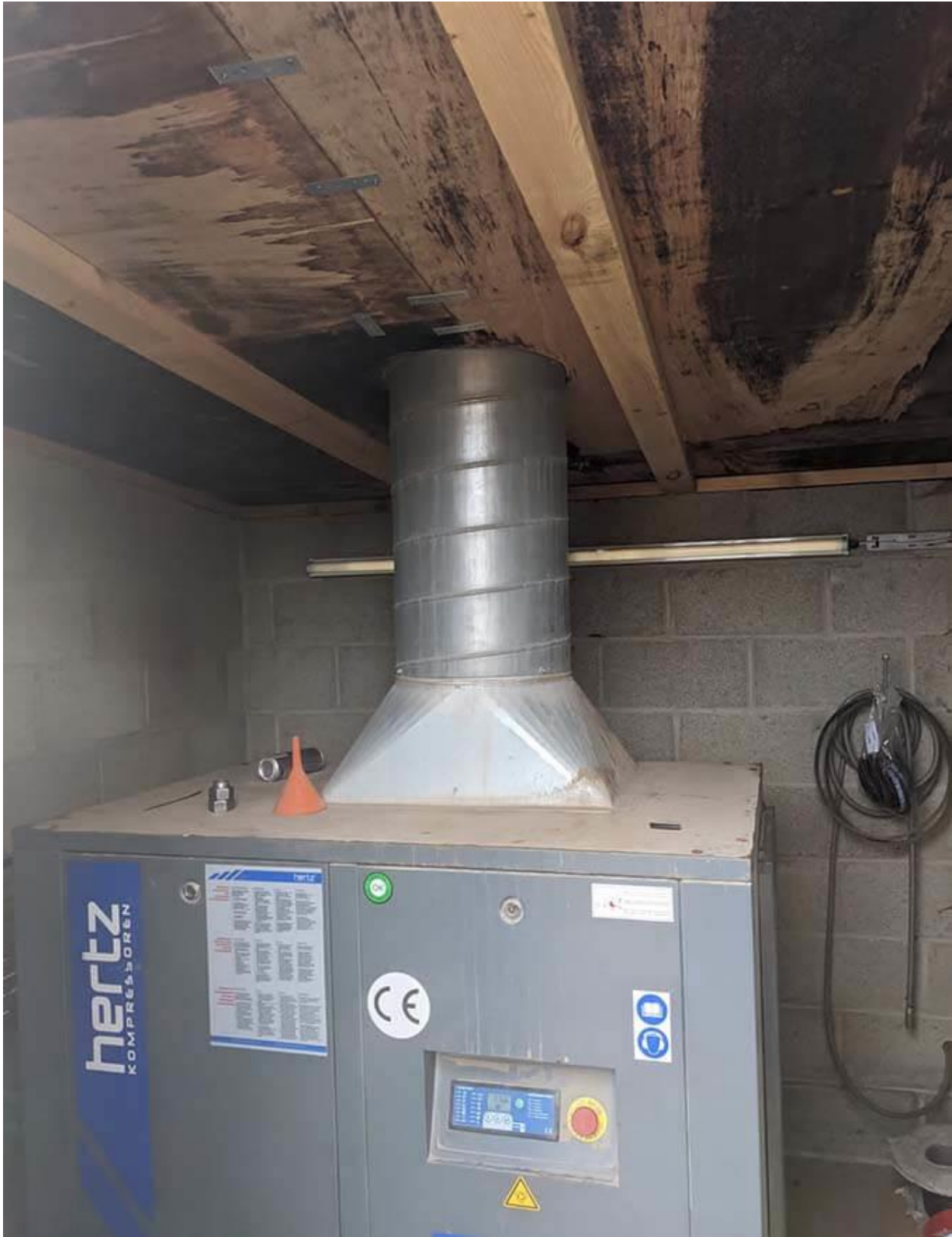
How quickly will a heat recovery system pay for itself?
