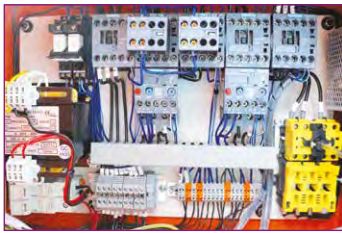
Clear-cut DC control cabinet
