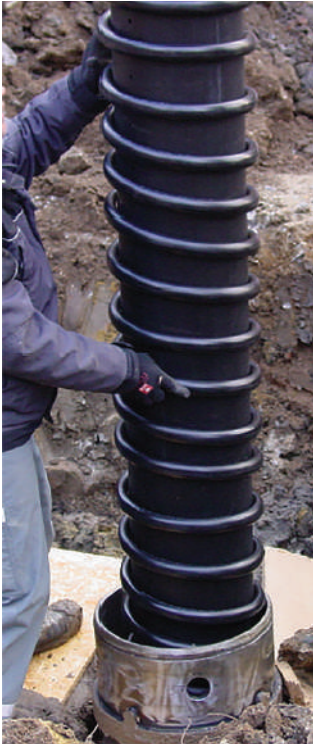
Installation by using a hollow auger drill
