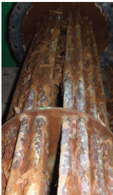
Scale on Heat Exchanger
