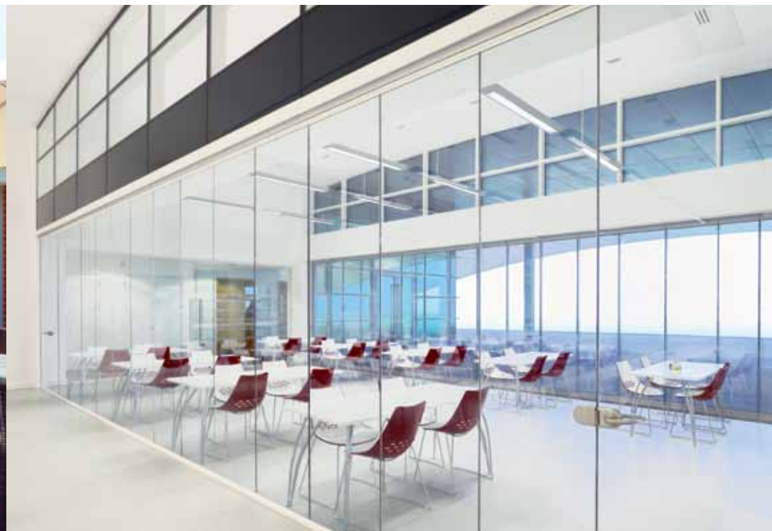
View of Manchester United's Trafford Centre staff restaurant looking through single-glazed curtains to restaurant extension with double-glazed curtains opening onto viewing area in the background
