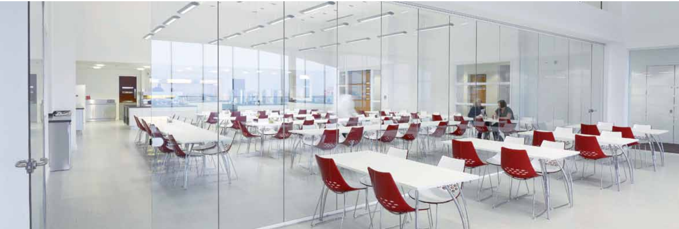
Recently completed installation at Manchester United's Trafford Centre staff restaurant. 18 single-glazed curtains each measuring 2.9m high x 0.8m wide
